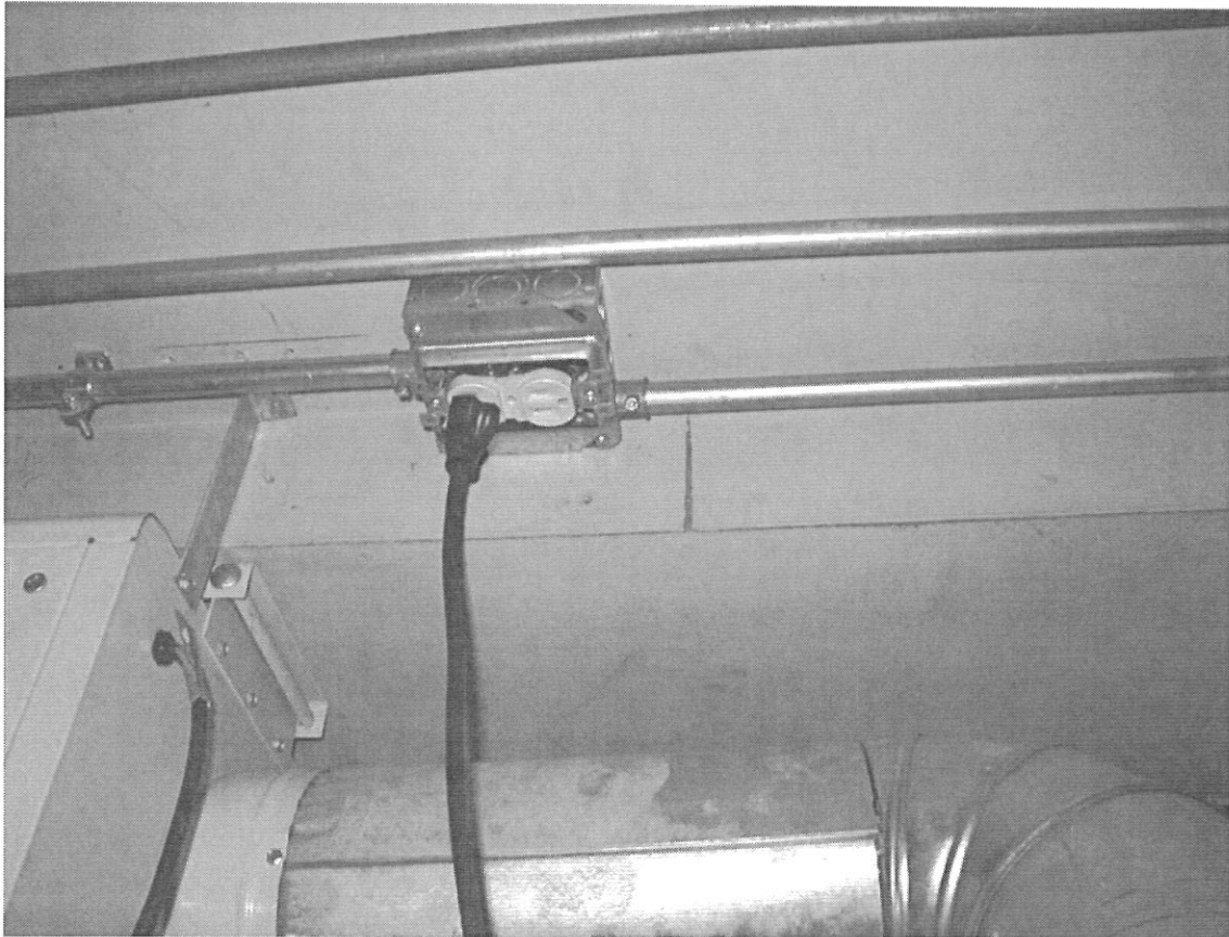
Missing Device Cover Plate
