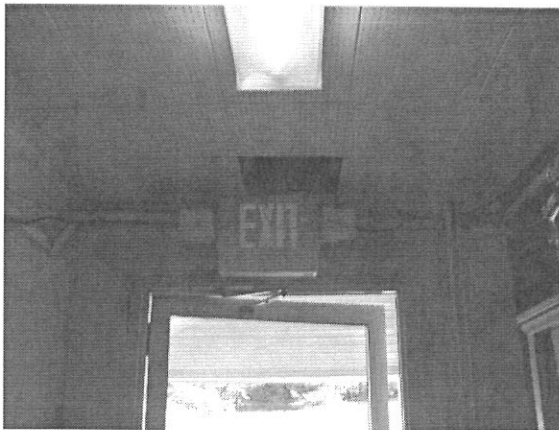
Combination Egress and Exit Lighting Unit
