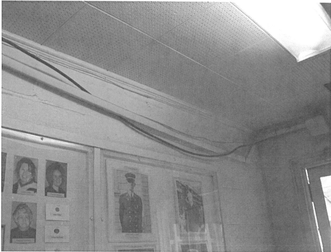
Telecom Pathways Improperly Supported
