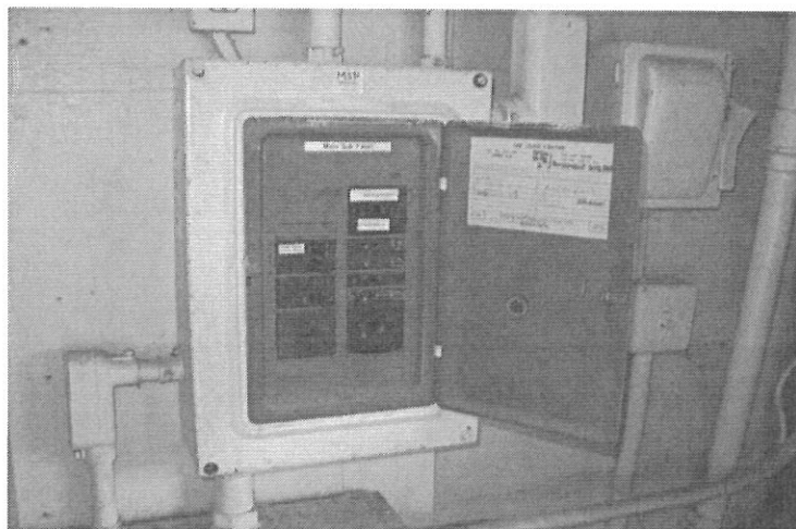
Sub-panel located in Vehicle Bay (Representative of a typical load center)
