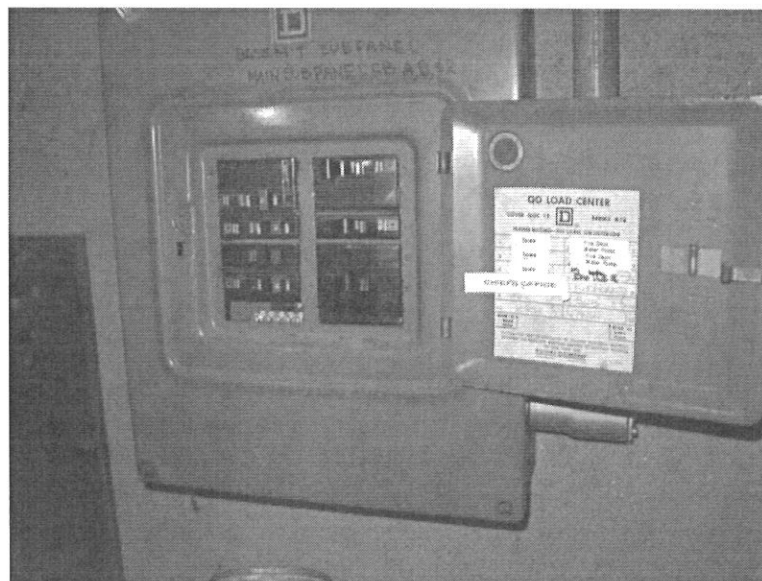
Note the New Labeling and Identification of Source Panel
