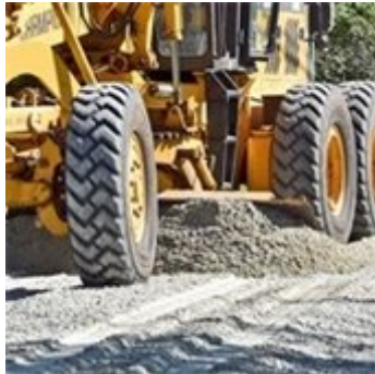
Summer road paving in Bow. Photo by Eric Anderson.
