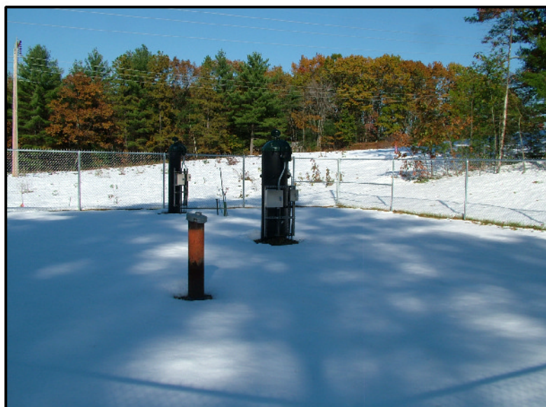
Production Wells PW-1 & PW-2 with Test Well in Foreground
