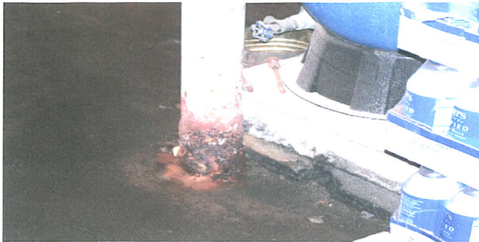
20. Rusted basement column, Fire Department
