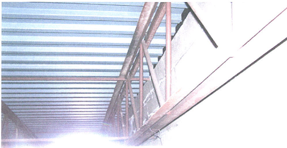
10. Interior Police Dept. Note: lack of diaphragm connection to wall.
