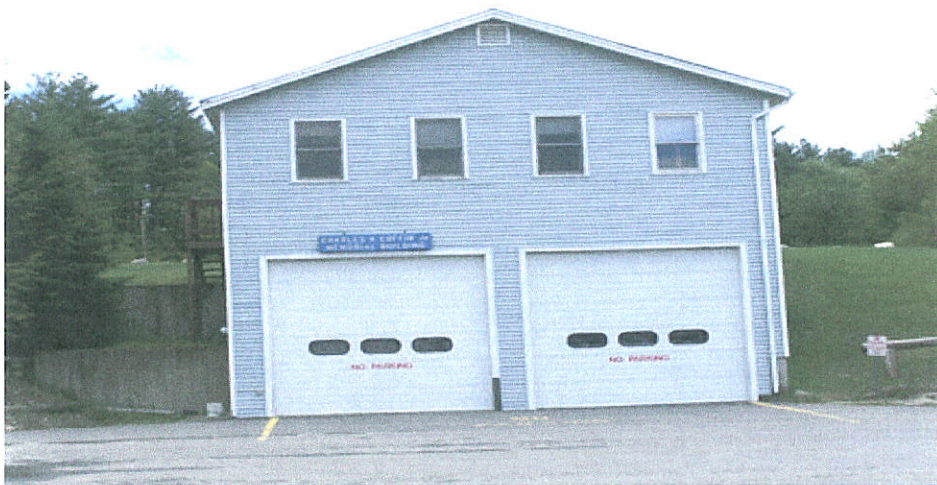
19. Bow Fire Dept., smaller building, Note: apparent lack of shear wall.
