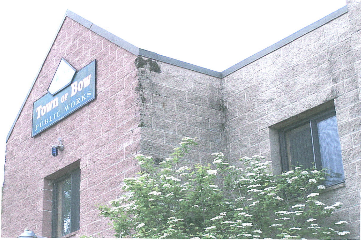
1. Police Station, Note: water stains and efflorescence
