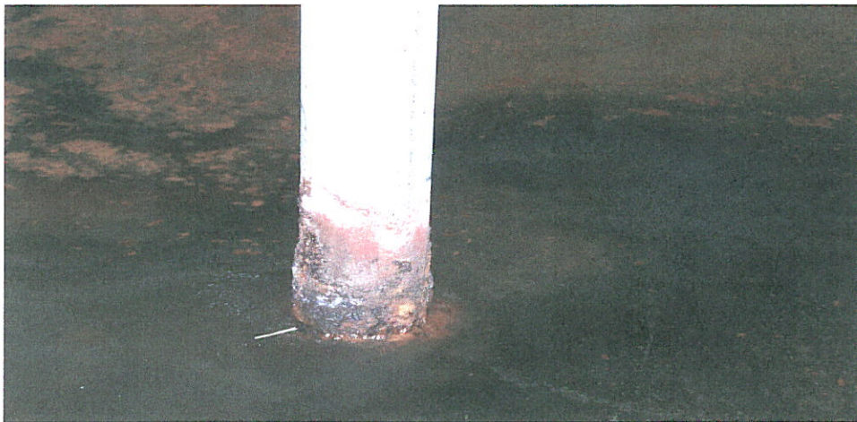
21. Rusted basement column Fire Department
